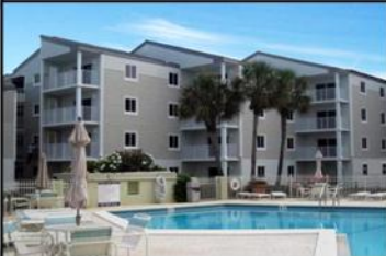
Sand Cliffs Restoration
